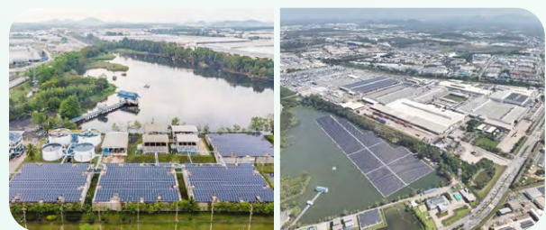
Eastern Seaboard Industrial Estate (Rayong) Water Reservoir
