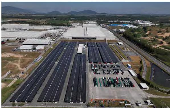
The solar power project for Ford Motor Company (Thailand) Limited, a global car manufacturing plant, is the largest Solar Car Park project in Thailand. It has a capacity of 7.7 MW, installed on the company’s parking lot area of 59,000 square meters. This installation will supply electricity to the company’s factory. This initiative will help reduce greenhouse gas emissions and electricity costs for customers, saving over 755 Million Baht over the project’s 25-year lifespan.
